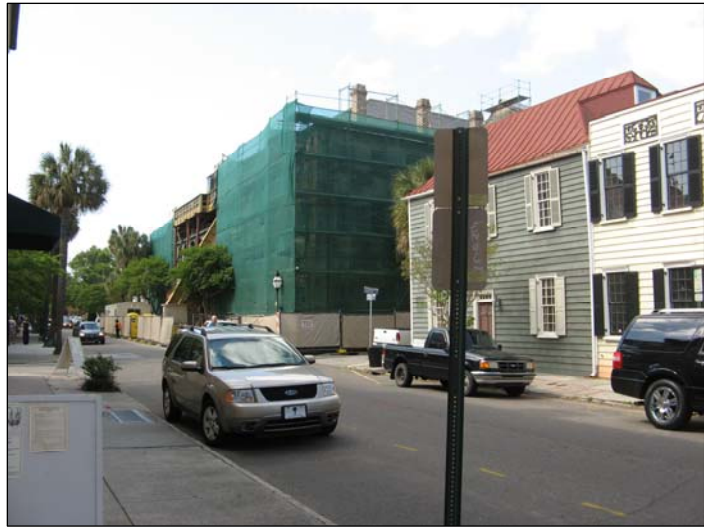
Figure 1: View of Dock Street structure, during renovation, facing southeast
