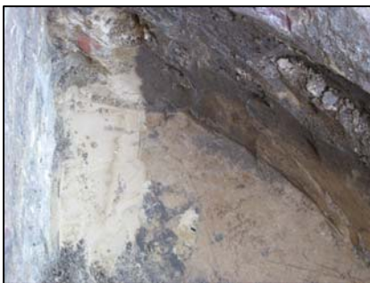
Figure 16: Drain (feature 5) and construction trench (feature 7) visible beneath the drain
